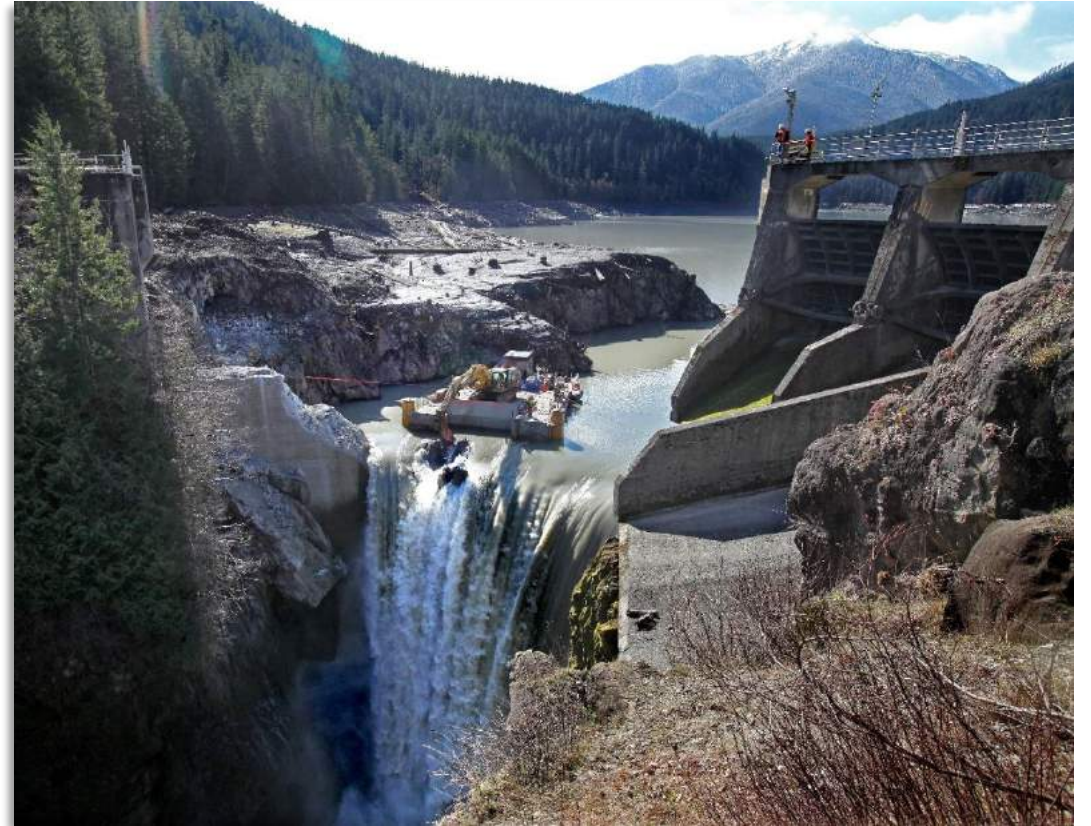
Glines Canyon Dam on the Elwha River
